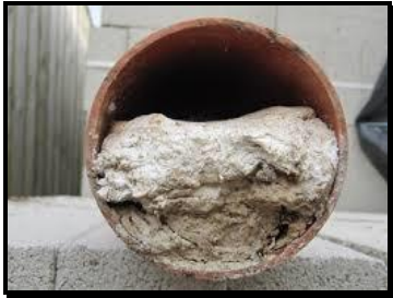
Grease clogging a sewer pipe
