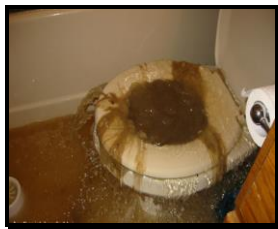
Sewer backing up through a toilet
